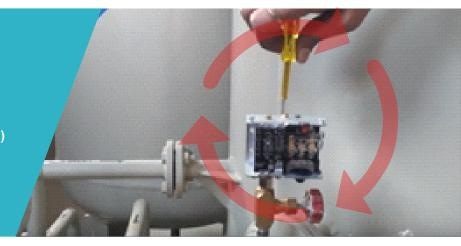
Put the lock cover back in position and screw it in place
