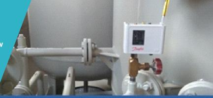
Turn the gas flow back on with the needle valve
