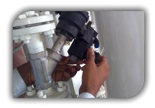
Open plunger housing by turning it in anti-clockwise direction with the help of adjustable wrench
