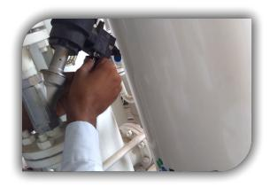
Close plunger housing by turning it in clock wise direction after fitting of plunger
