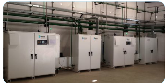
2 Nos. 30 Nm 3 /hr Hydrogen Generators in Karnataka at world's largest MIM part manufacturer
