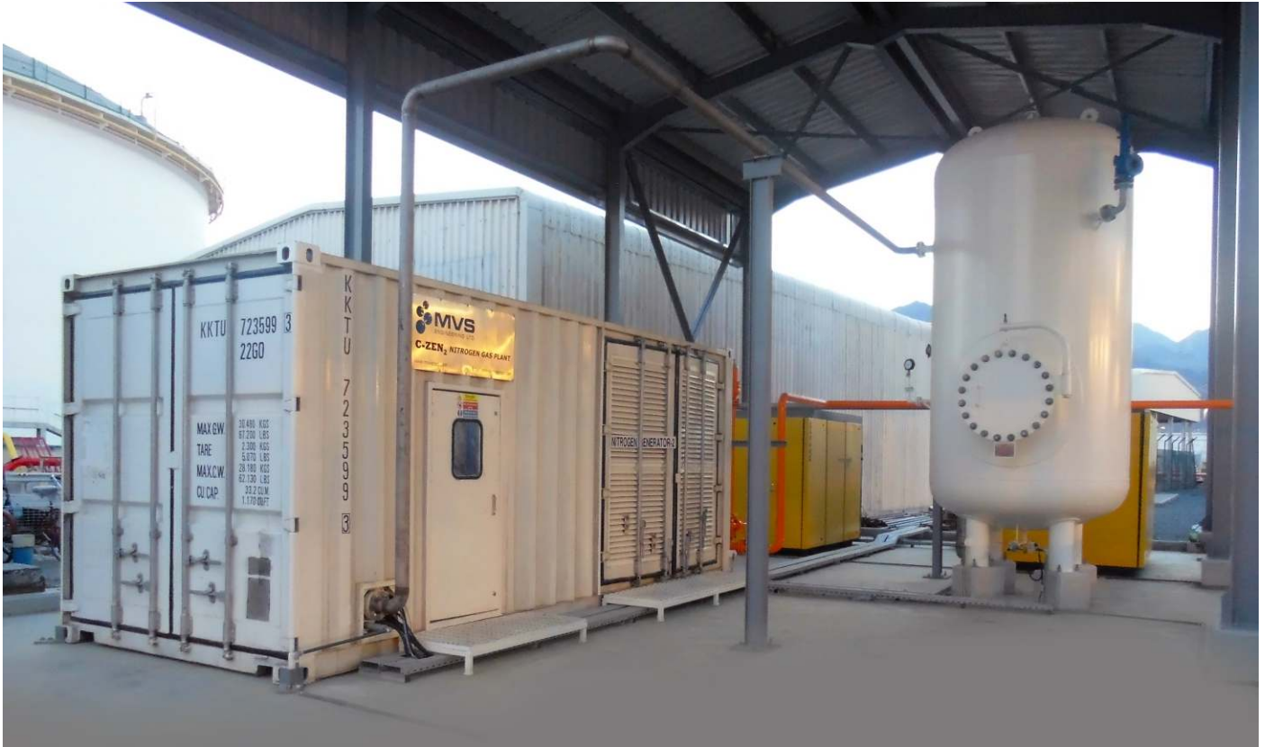
C-ZEN Containerized Units with integrated compressor. 300 Nm 3 /hr Nitrogen flow for Petrochemical Tanks and Oil Field application
